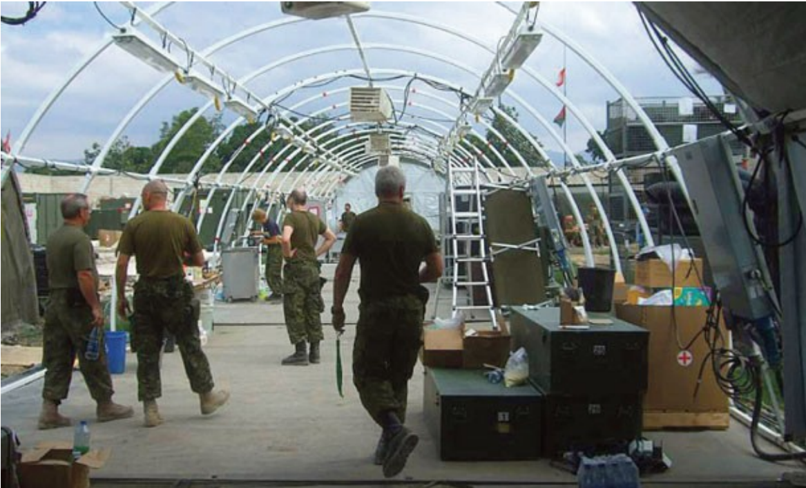
Tear down of the 1 Canadian Field Hospital deployed in Haiti.
